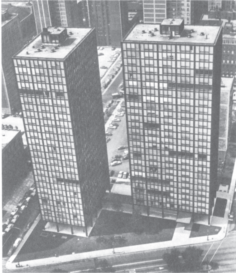
Figure 21 860–880 Lake Shore Drive, Chicago, USA: apartment blocks designed by Mies van der Rohe. Hedrick-Blessing photograph, courtesy Chicago Historical Society.
