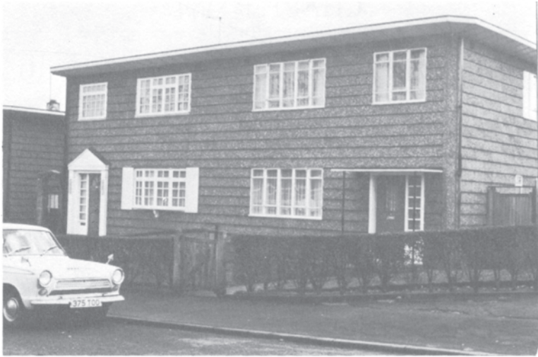
Figure 1 1950s semi-detached house in East London, precast concrete system-built. The house on the left has been modified by its occupant.
