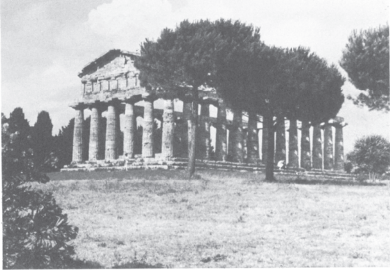
Figure 17 Greek Temple in Paestum, Italy. Note the construction of the columns: the blocks are fluted, which camouflages their assembly sequence of one block placed upon another.
