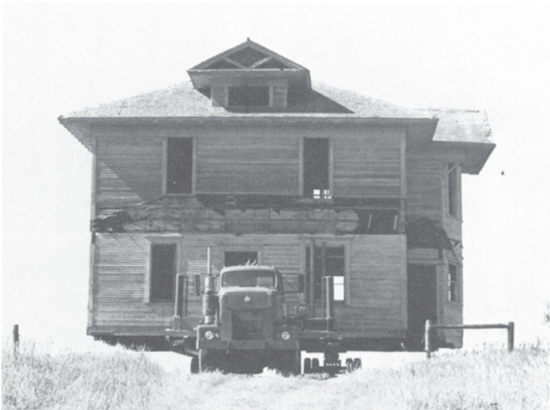
Figure 5 Moving house. This activity places unusual loads on the structure. Photo © Sally and Richard Greenhill.
