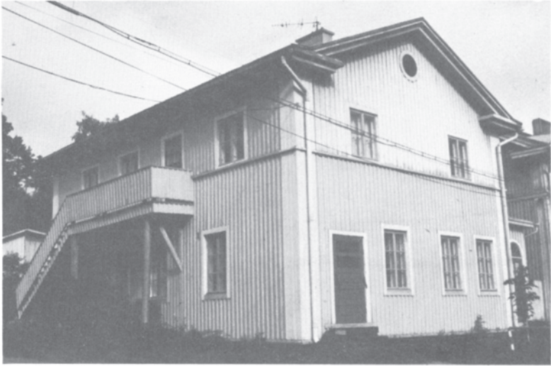
Figure 39 House, Jyväskylä, Finland: designed by Alvar Aalto. Note the timber detail—cover batten over vertical butt-joints, giving a 'corduroy' or 'reversed fluting' effect.
