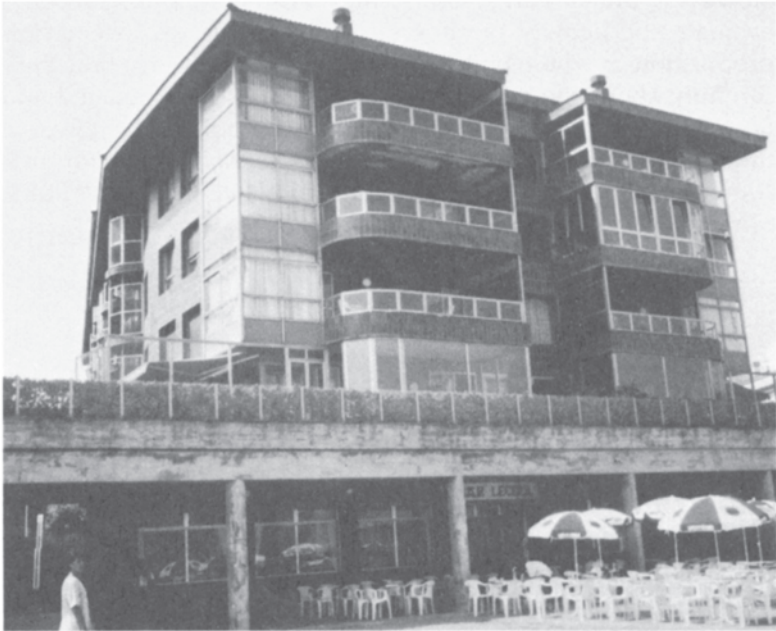
Figure 9 Seaside block: building on the North Spanish coast. Note the complex system of glazed and open balconies, providing control of wind, solar radiation, heat loss, etc.
