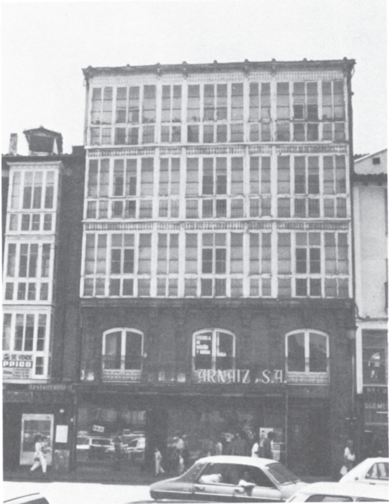
Figure 8 Urban block: buildings in Bilbao, Spain. Note the use of a glazed volume outside the door/windows of the buildings. This enables a complex control system of solar radiation, heat loss, ventilation, etc.
